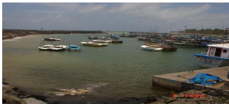
Vessels anchored in the limited space in the Harbour Basin
