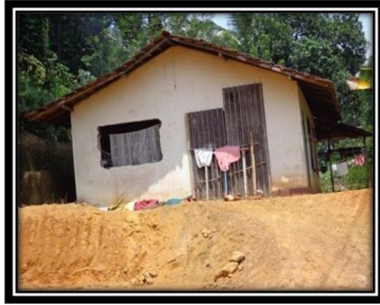
Photograph 6 House of an evacuated Family
