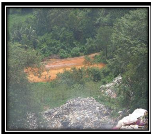
Photograph 4 Landslide of the Garbage Heap
