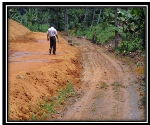
Photograph 5 Reconstruction of the Road and Construction of the Earth Bund
