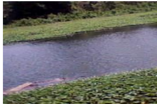
Obstruction caused to main channels by Water Hyacinth observed at field inspections in Polonnaruwa District
