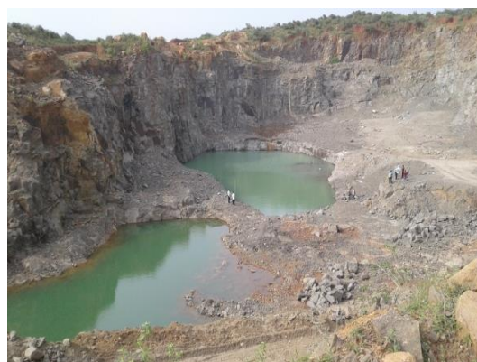
Diagram 26 - Unauthorized quarry in the middle of the proposed southern express way at CH8+250-500 k.m. ( The depth of the quarry was 28 meters as per the measurements of the Department of Surveyor General)
