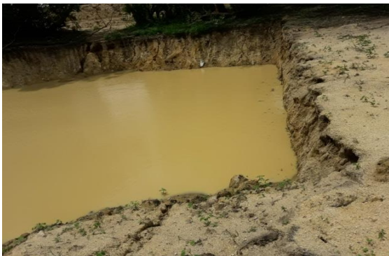
Figure 11 - How Bogoda tank have been dug and dug beyond the permitted depth
